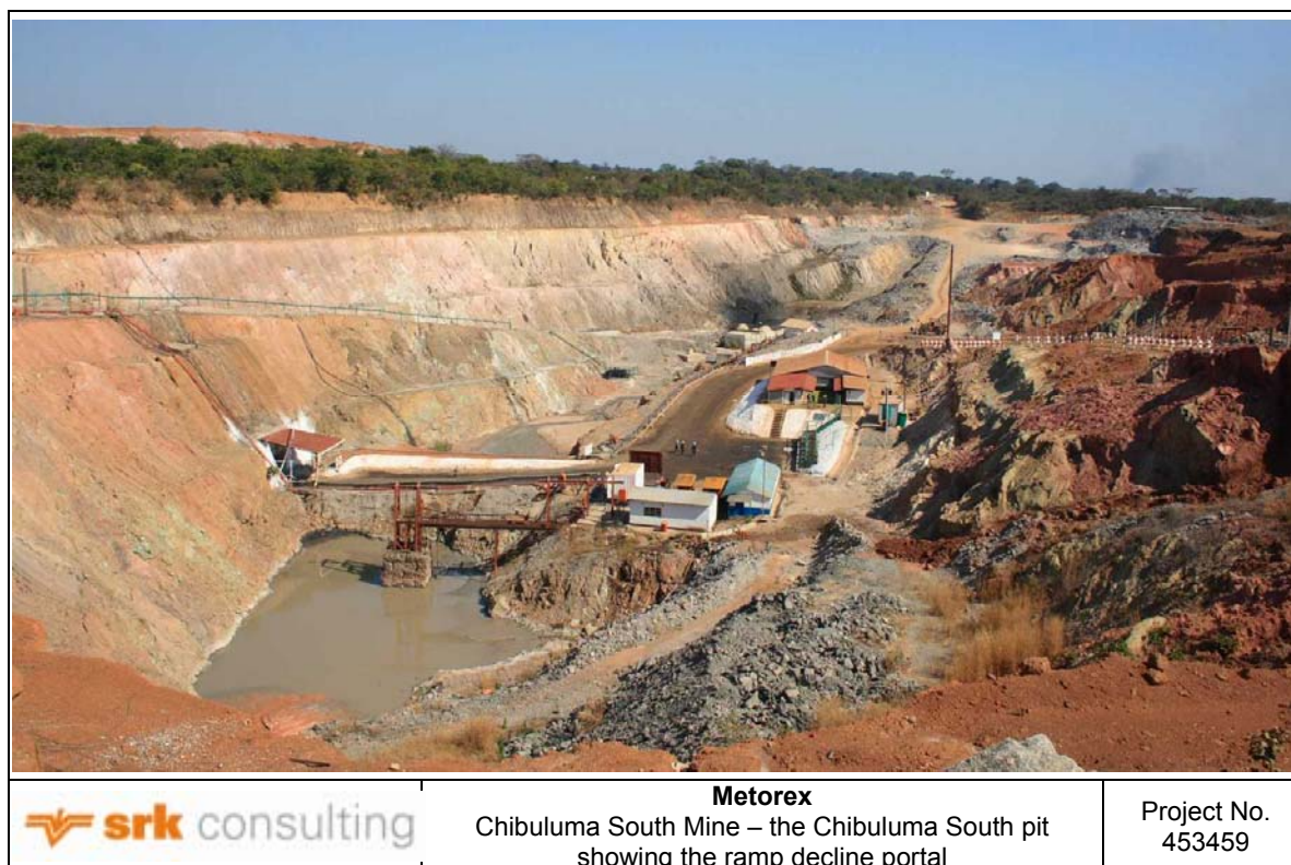
Figure 4.15: Chibuluma South Mine – the Chibuluma South pit showing the ramp decline portal
